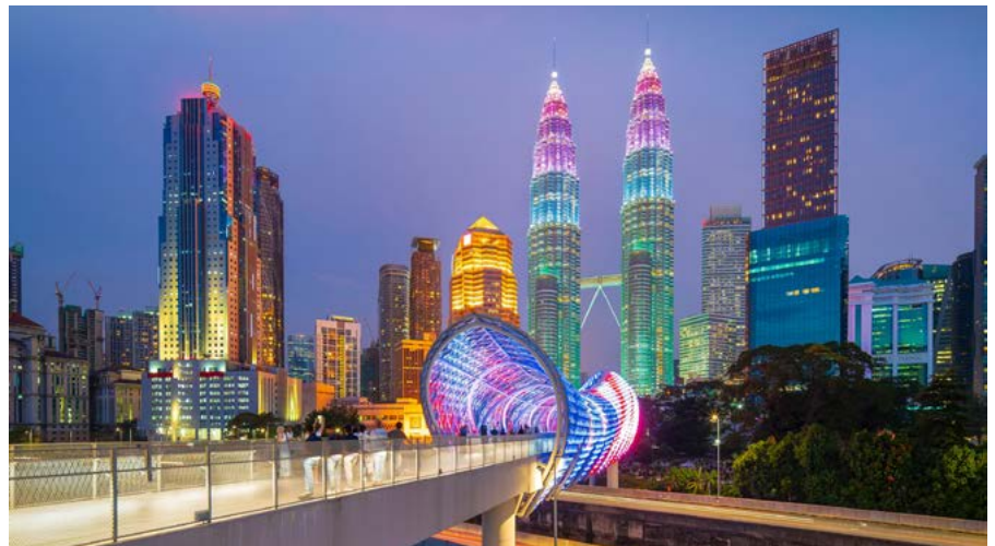
Saloma Link Bridge, Kuala Lumpur
