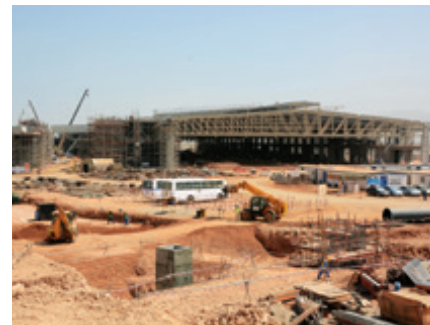
Oman Convention Center under construction
