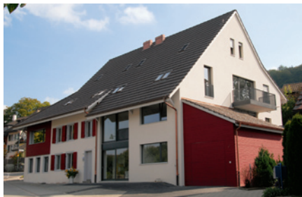
New office building in Lupsingen (on ground level) at Seltisbergerstrasse 16
