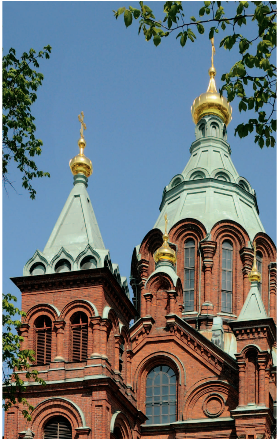
Uspensky Orthodox Cathedral, Helsinki, completed in 1868
