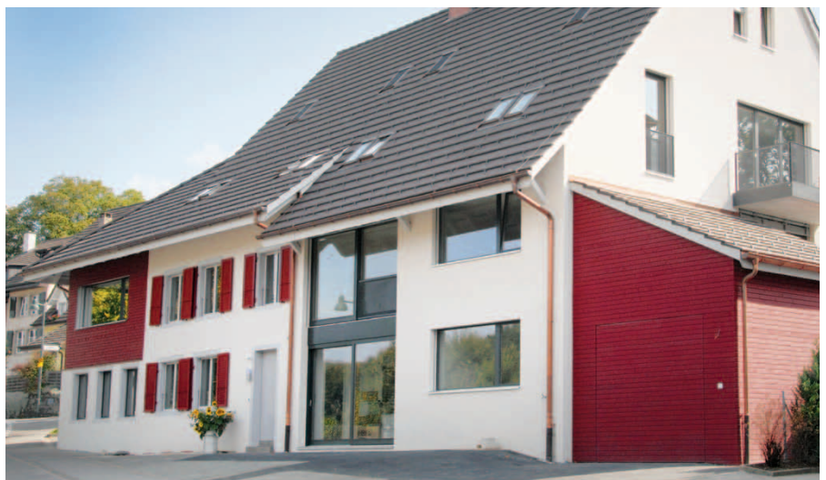
ISS/SIC Office Building (Ground Level) at Seltisbergerstrasse 16 in Lupsingen nearby Basel, Switzerland
